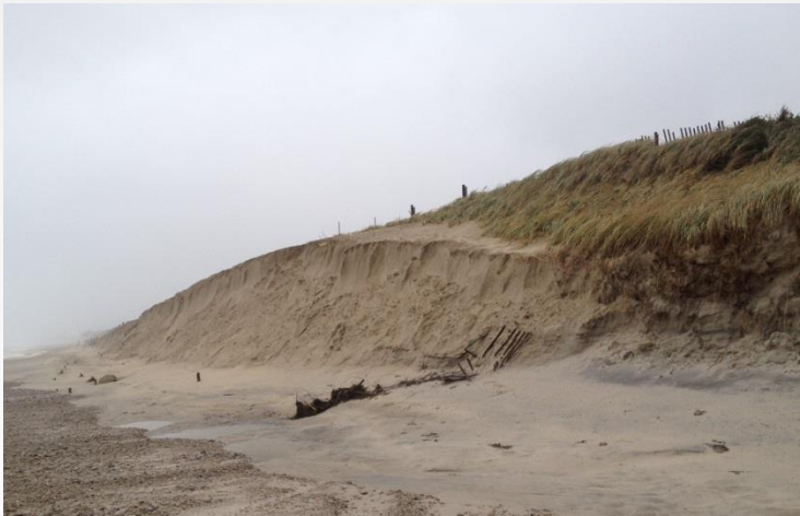
Primary dune looking east 1 month prior to 2 nd emergency sand placement in December 2014.
