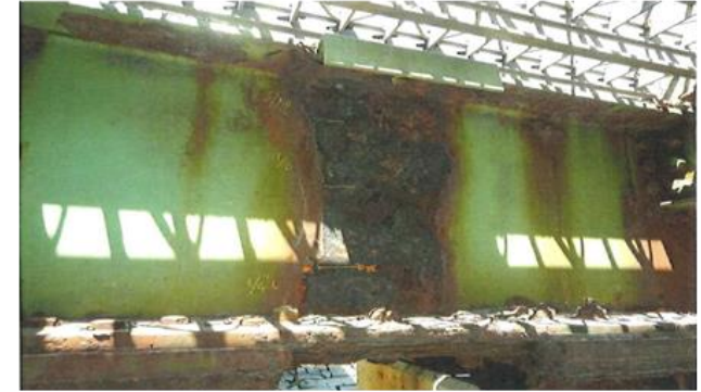
North Bay Bridge severe corrosion
