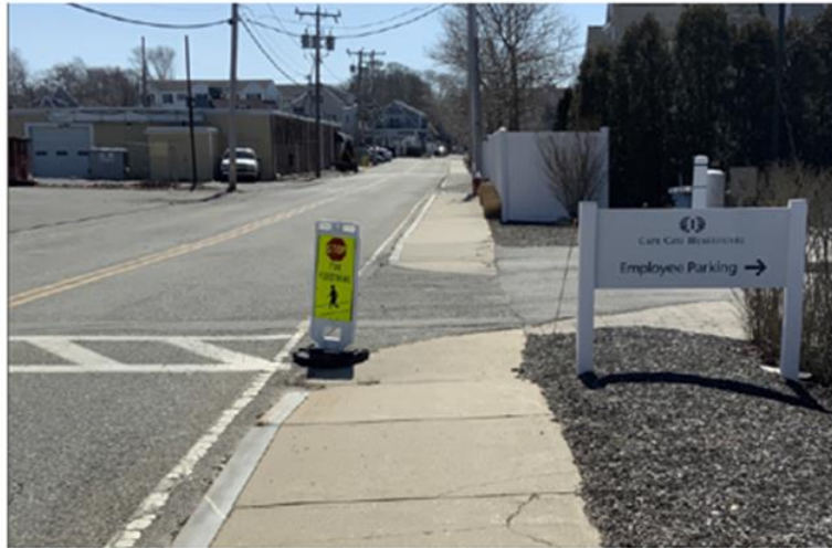
Exceeds allowable cross-slope pitch
