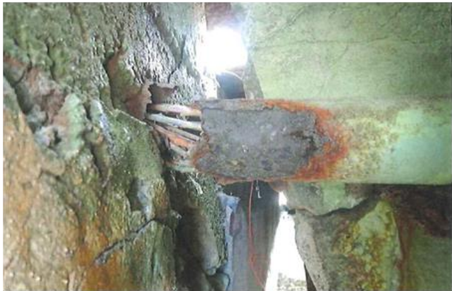
North Bay Bridge exposed wires
