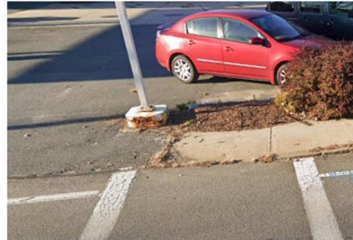
Missing detectable warning
