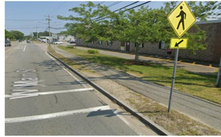
Missing curb ramp
