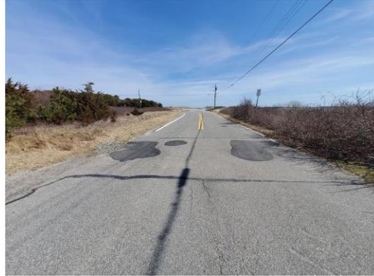
Asphalt and rock patches on Hawes Avenue due to broken culvert pipe under roadway (taken 3-15-2022).
