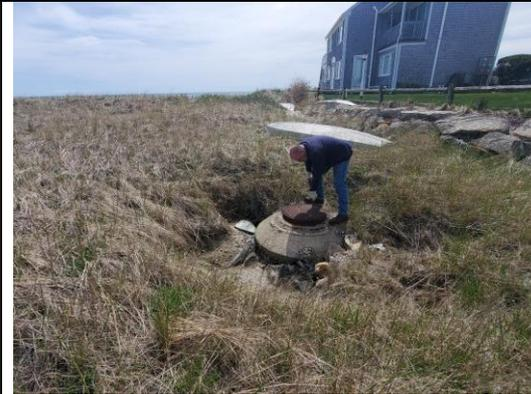
Junction manhole at the connection of an older culvert to a newer culvert that allows salt water connection to the upgradient salt marsh (taken 3-15-22).
