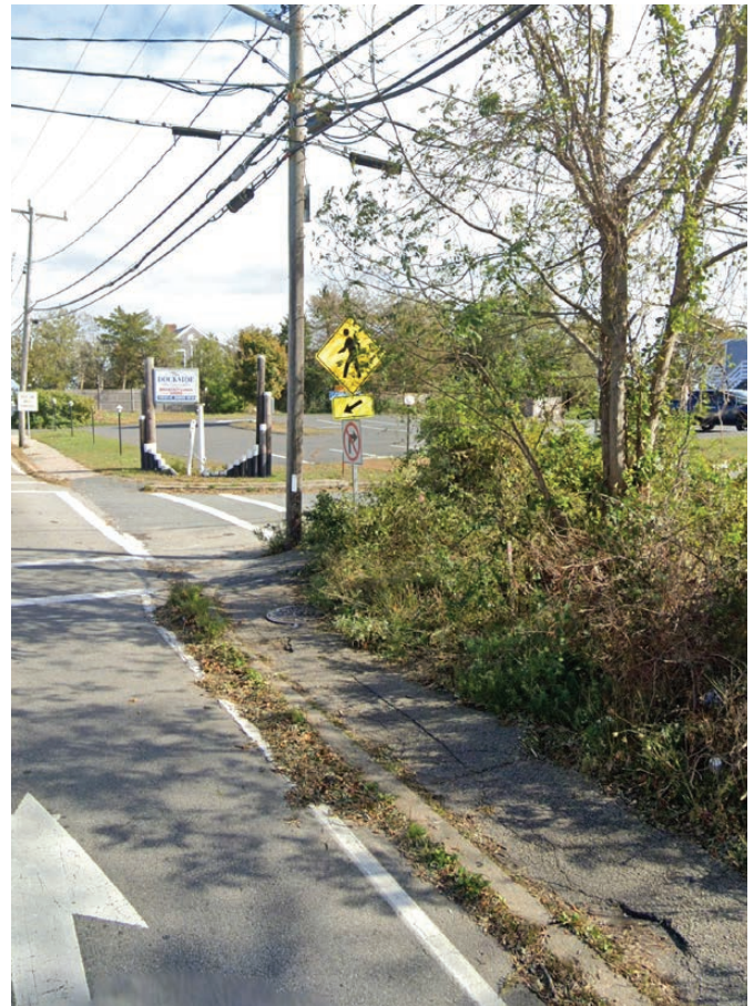
Figure 26: Overgrown Sidewalks on South Street, looking east Source: Google Earth, 2024
