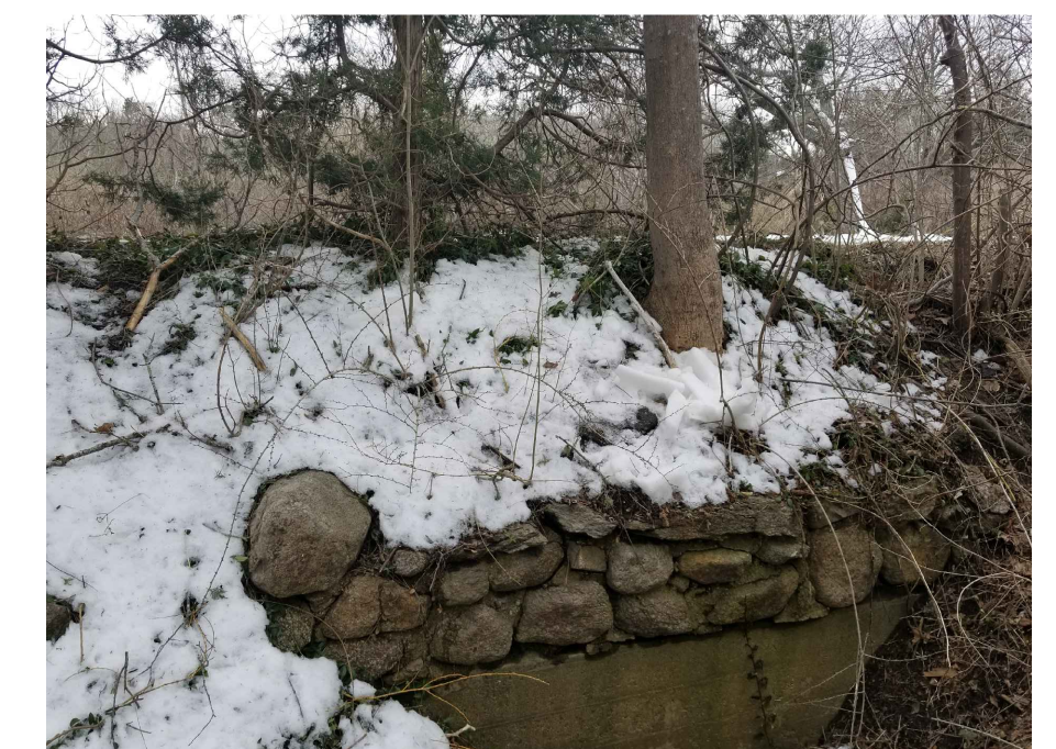
PHOTO 4 EXISTING DOWNSTREAM CULVERT, VIEW LOOKING SOUTH
