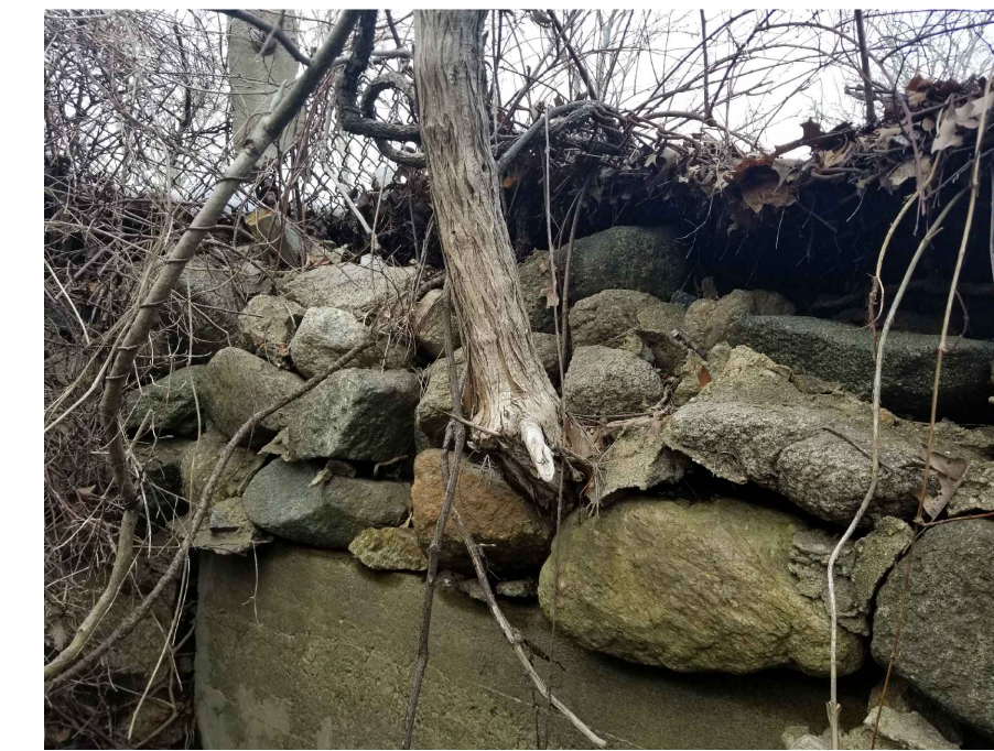
PHOTO 2 STONE/EARTH RETAINING WALL ABOVE UPSTREAM CULVERT, VIEW LOOKING NORTH
