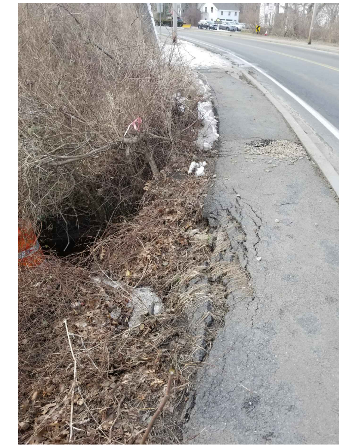
PHOTO 1 EXISTING SIDEWALK LOOKING DOWN AT CULVERT, VIEW LOOKING WEST
