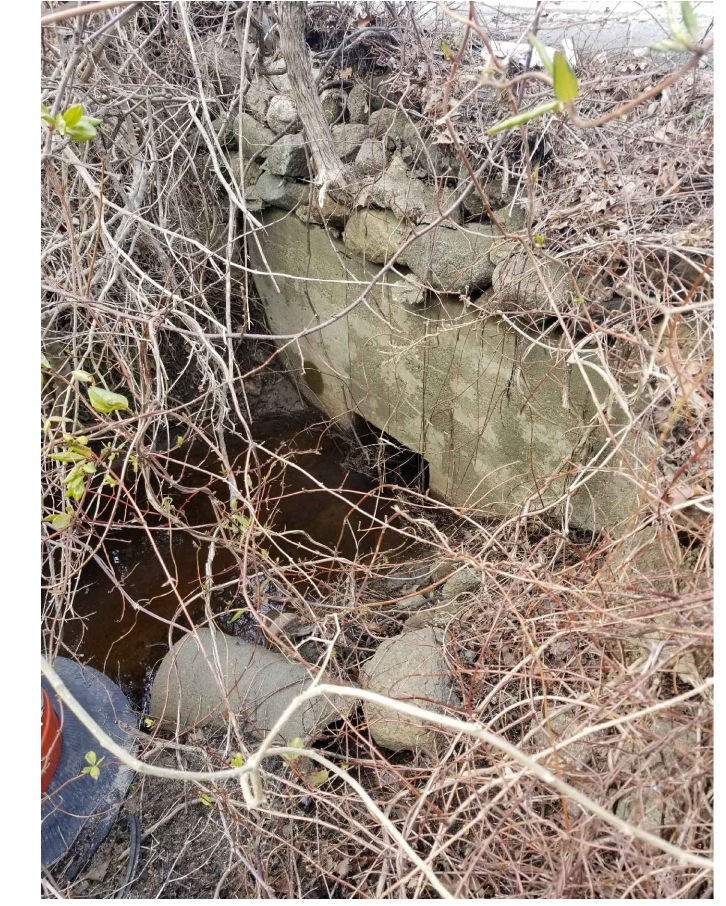
PHOTO 3 EXISTING UPSTREAM CULVERT, VIEW LOOKING NORTH
