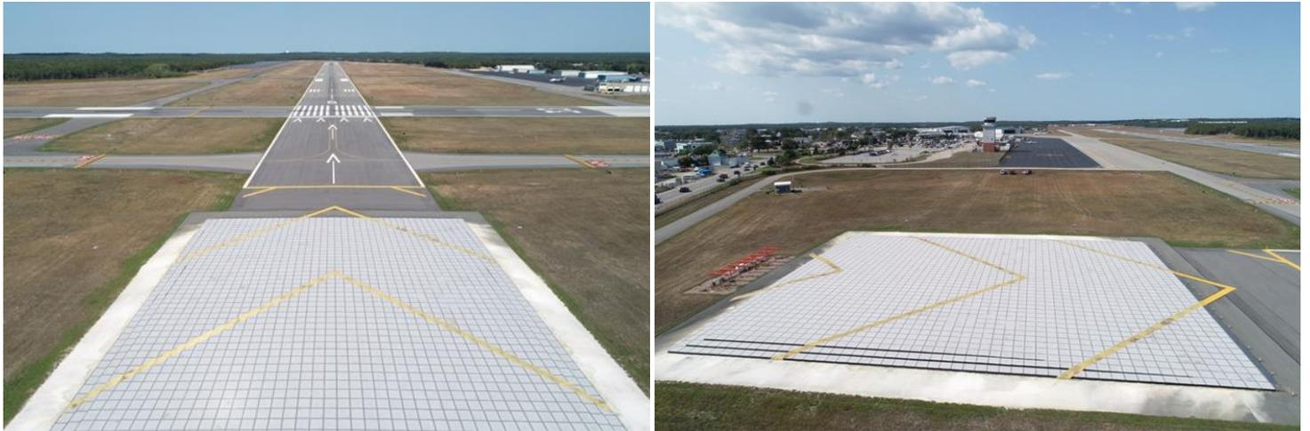
Engineered Materials Arresting System (EMAS)
