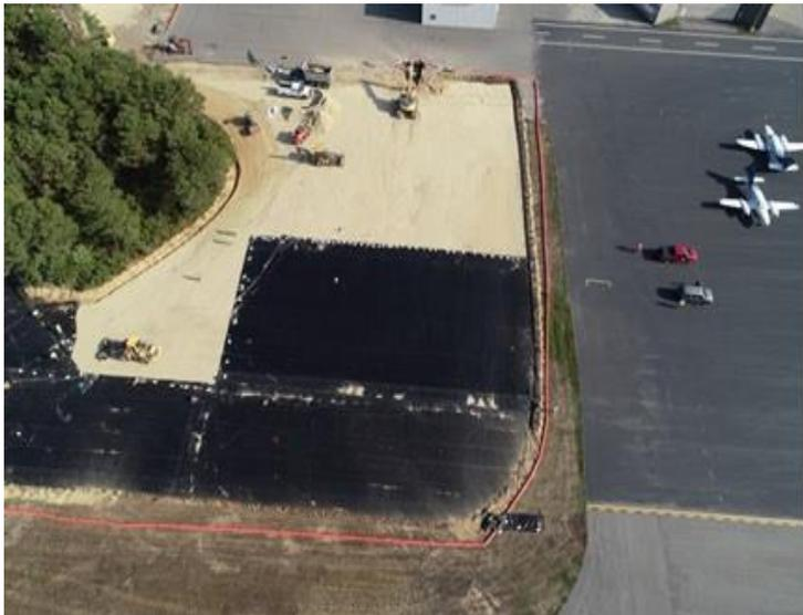
Photo shows excavated PFAS impacted soils removed and installation of a poly-fiber cap as a permanent solution for mitigation.
