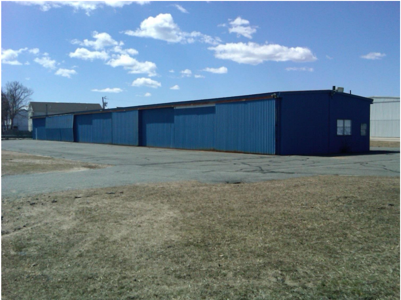
Airport-owned Existing T-hangar
