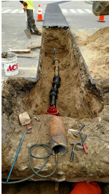
Water Pipe Replacement
