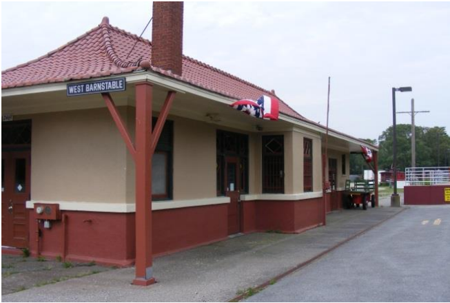
West Barnstable Railroad Depot
