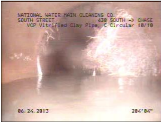
Sewer Pipe Root Intrusion
