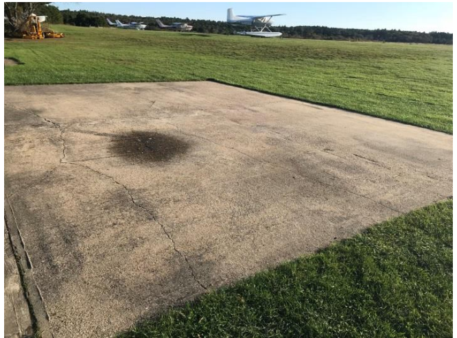
Cape Cod Air Field Underground Fuel Tank
