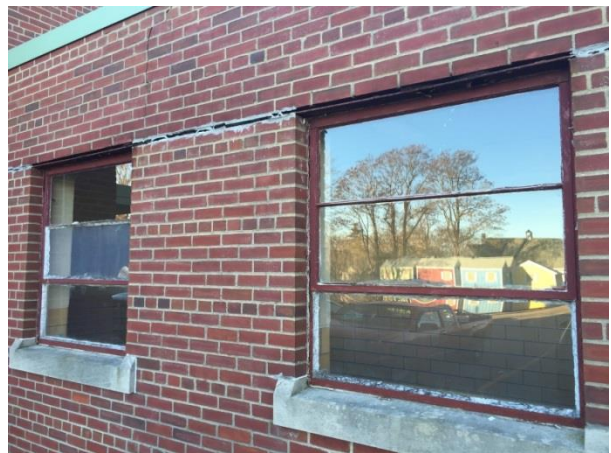
Armory Building Exterior
