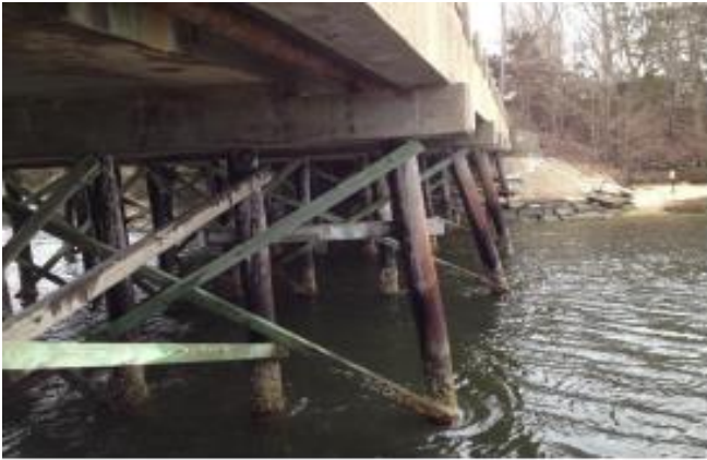
Bumps River Bridge
