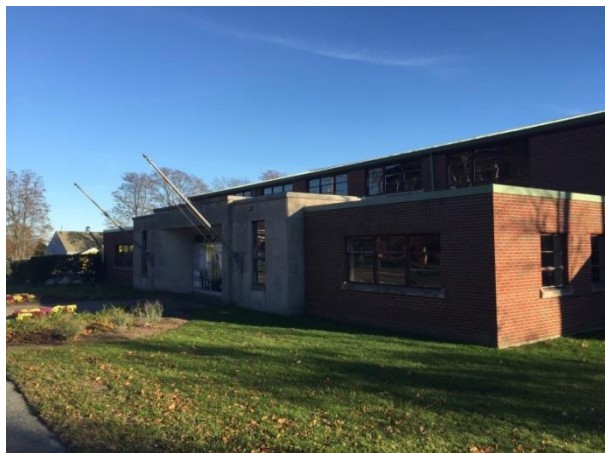
Armory Building Exterior
