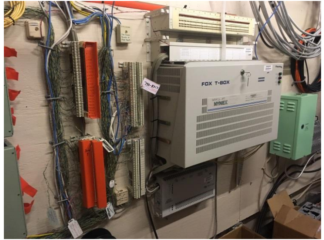
Existing High School Demark
