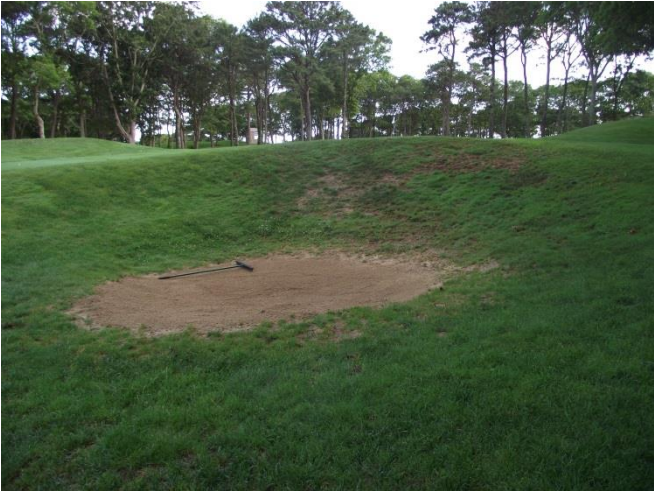
Hole #2 Deteriorating Bunker
