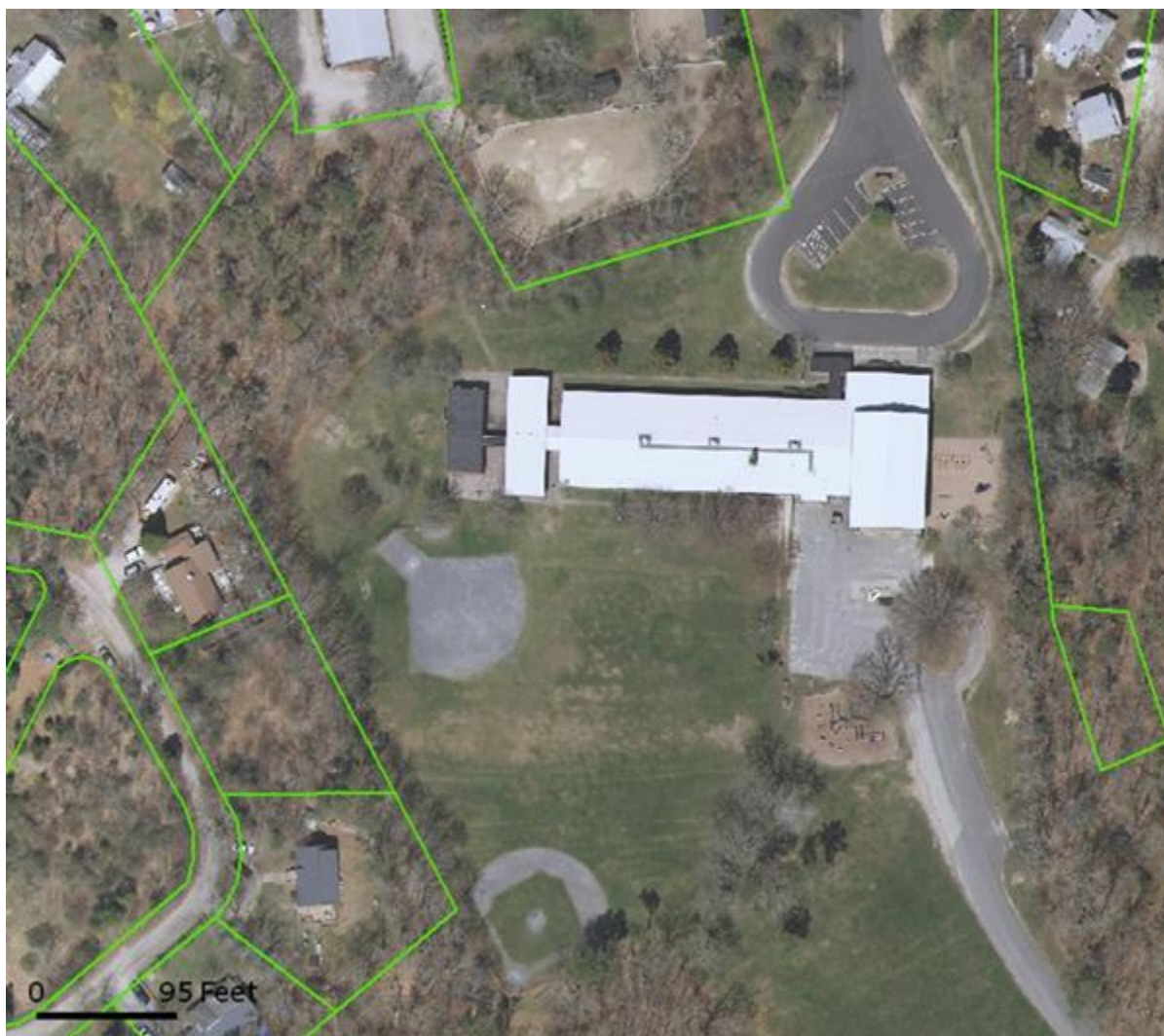
Marston Mills Elementary School (Closed in 2010) to be demolished
