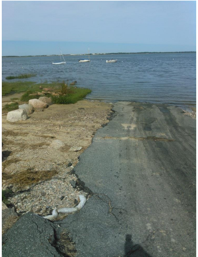
Scudder's Lane Boat Ramp
