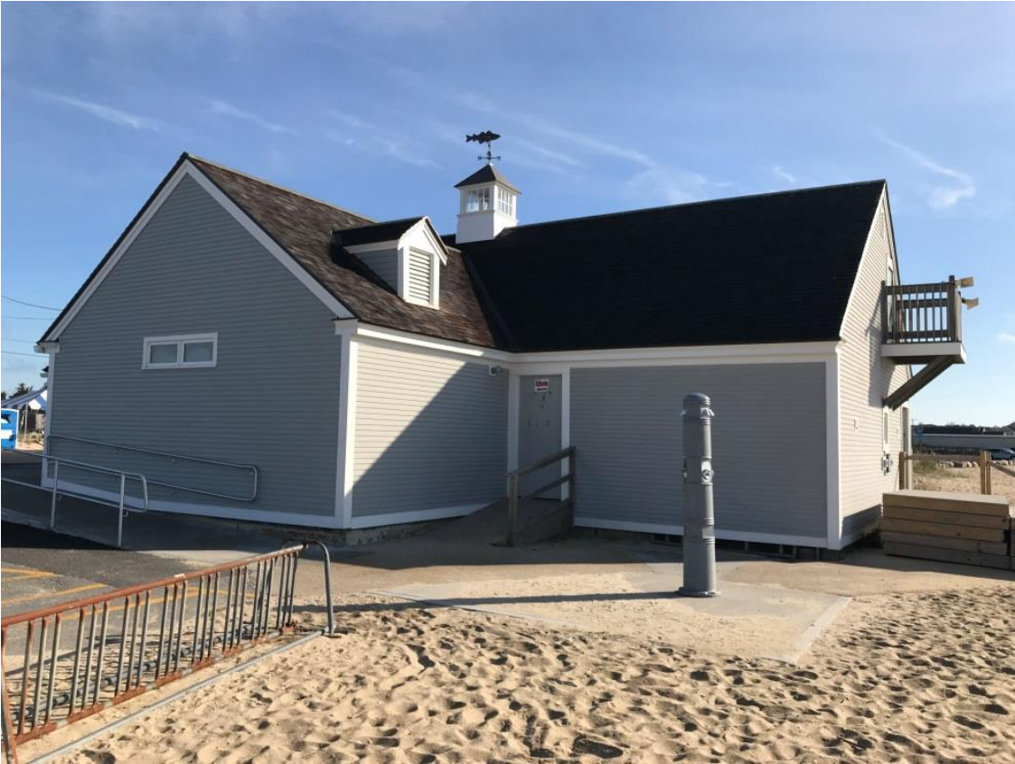
Craigville Bathhouse Septic Location
