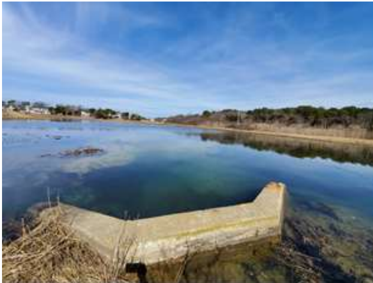
Culvert headwall and up-gradient salt marsh (taken 3-15-22).
