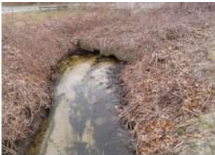
Culvert under Lake Elizabeth Drive (Restriction 1)
