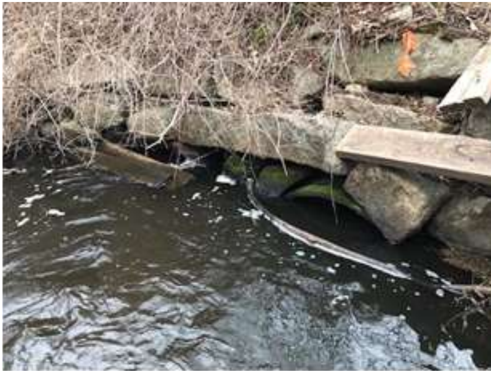
Photo 1: Looking at culvert (nearly underwater) on upstream side of Rosa Lane.
