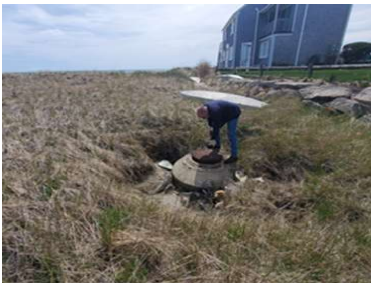
Junction manhole at the connection of an older culvert to a newer culvert that allows salt water connection to the up gradient salt marsh (taken 3-15-22).
