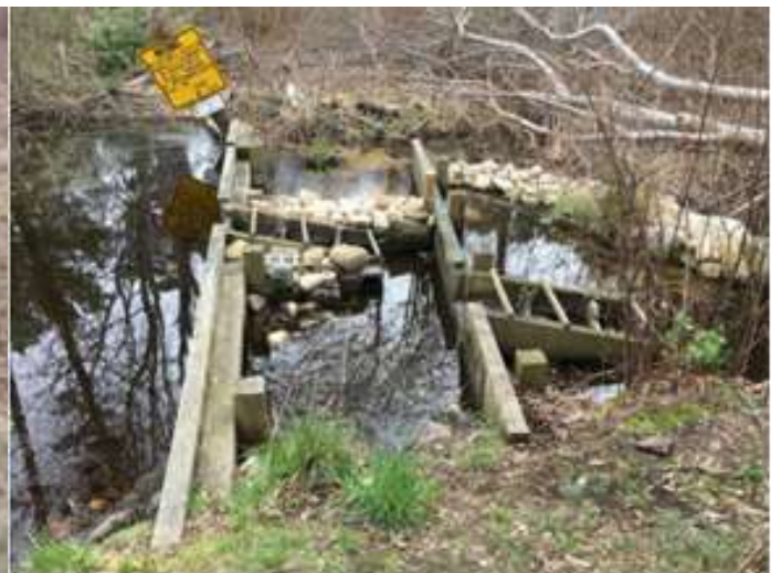
Fish Ladder/Dam at Lake Elizabeth (Restriction 2)
