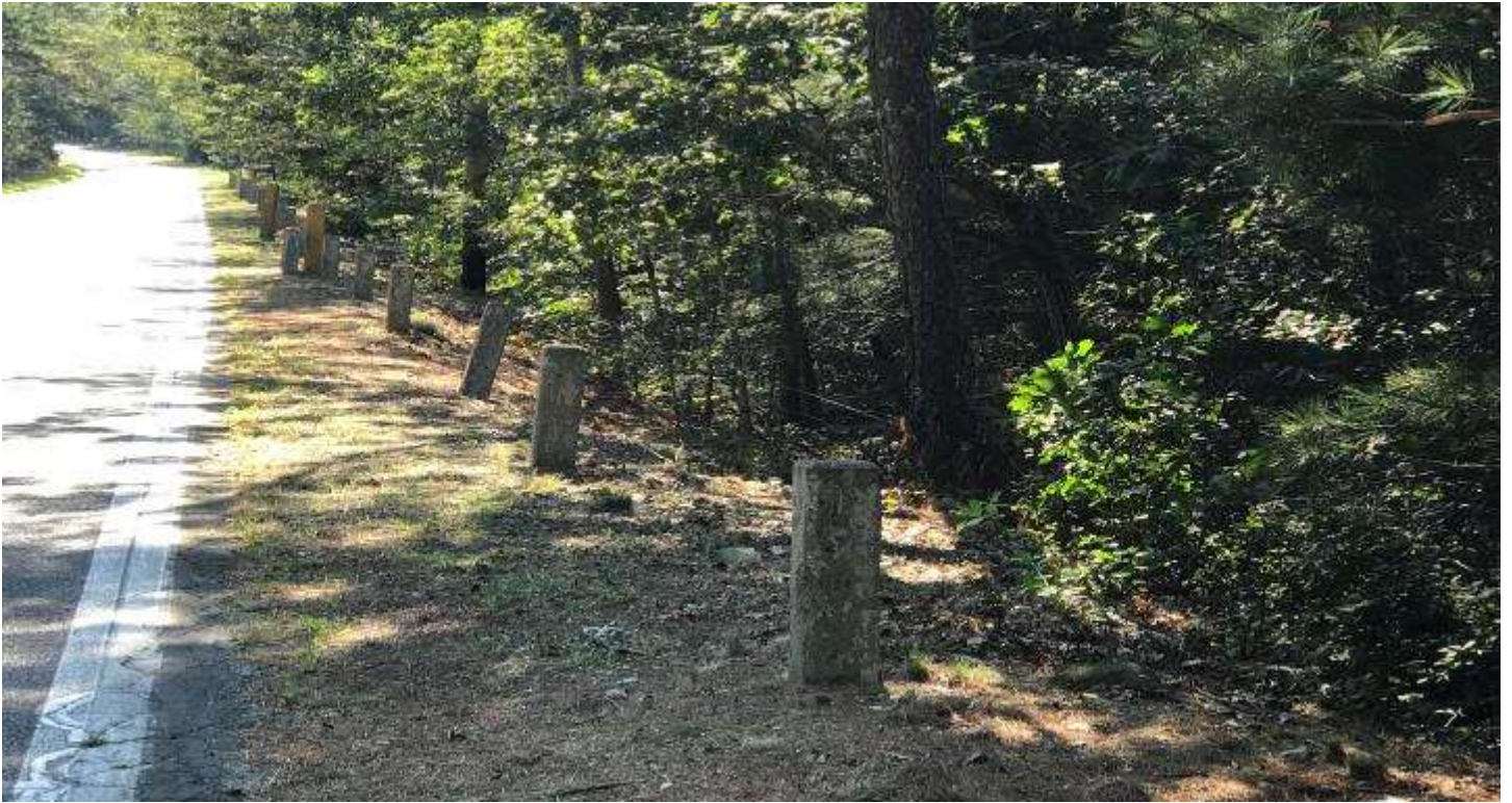
Concrete Guardrail Removal
