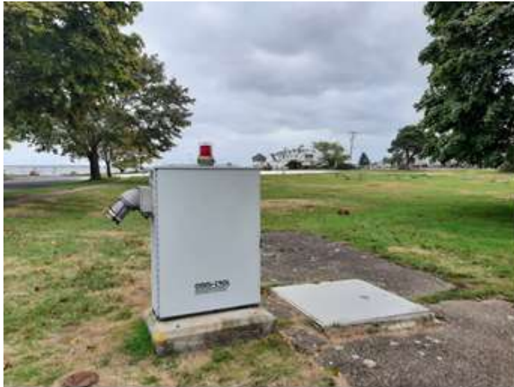
Photo 3: Gosnold Street Pump Station
