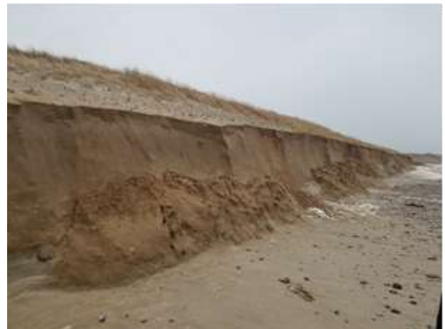
Post Storm Dune Erosion
