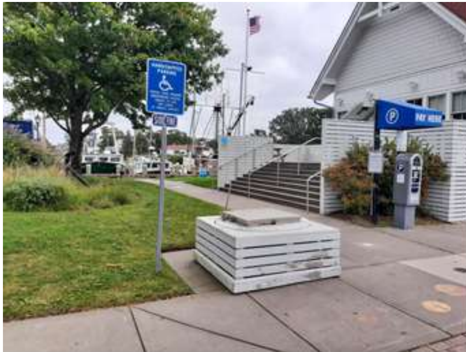
Photo 1: Ocean Street Pump Station
