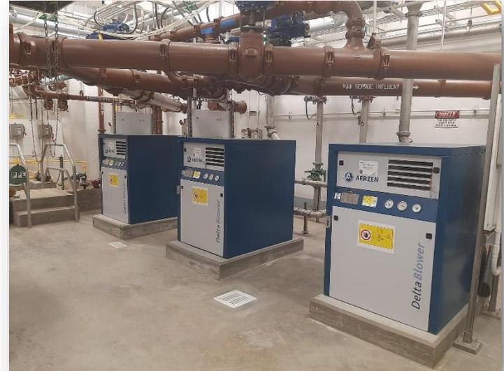
*New blowers used for mixing sludge tanks*
