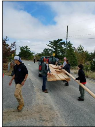
Unloading the wood and getting ready for the project.
