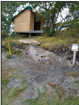
This is the current condition after the busy day! More work needs to be done to complete the project and everyone will be told the next date.
