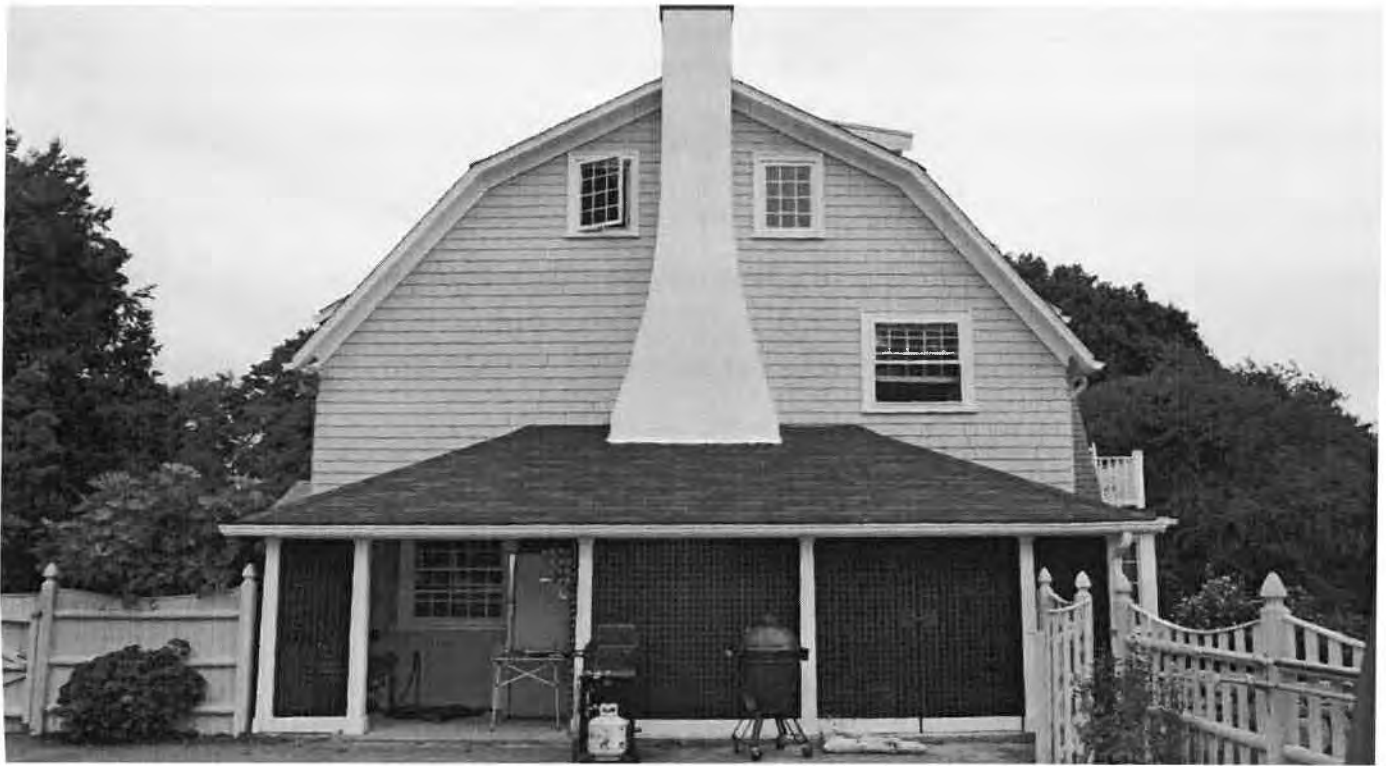
VIEW OF WEST ELEVATION (RIGHT FROM FRONT)
