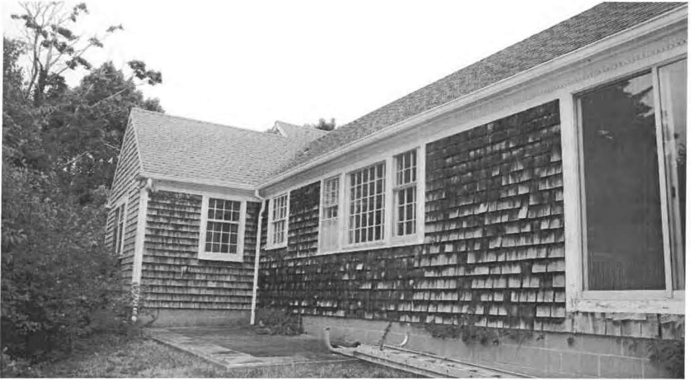
VIEW OF EAST ELEVATION (RIGHT FROM FRONT)
