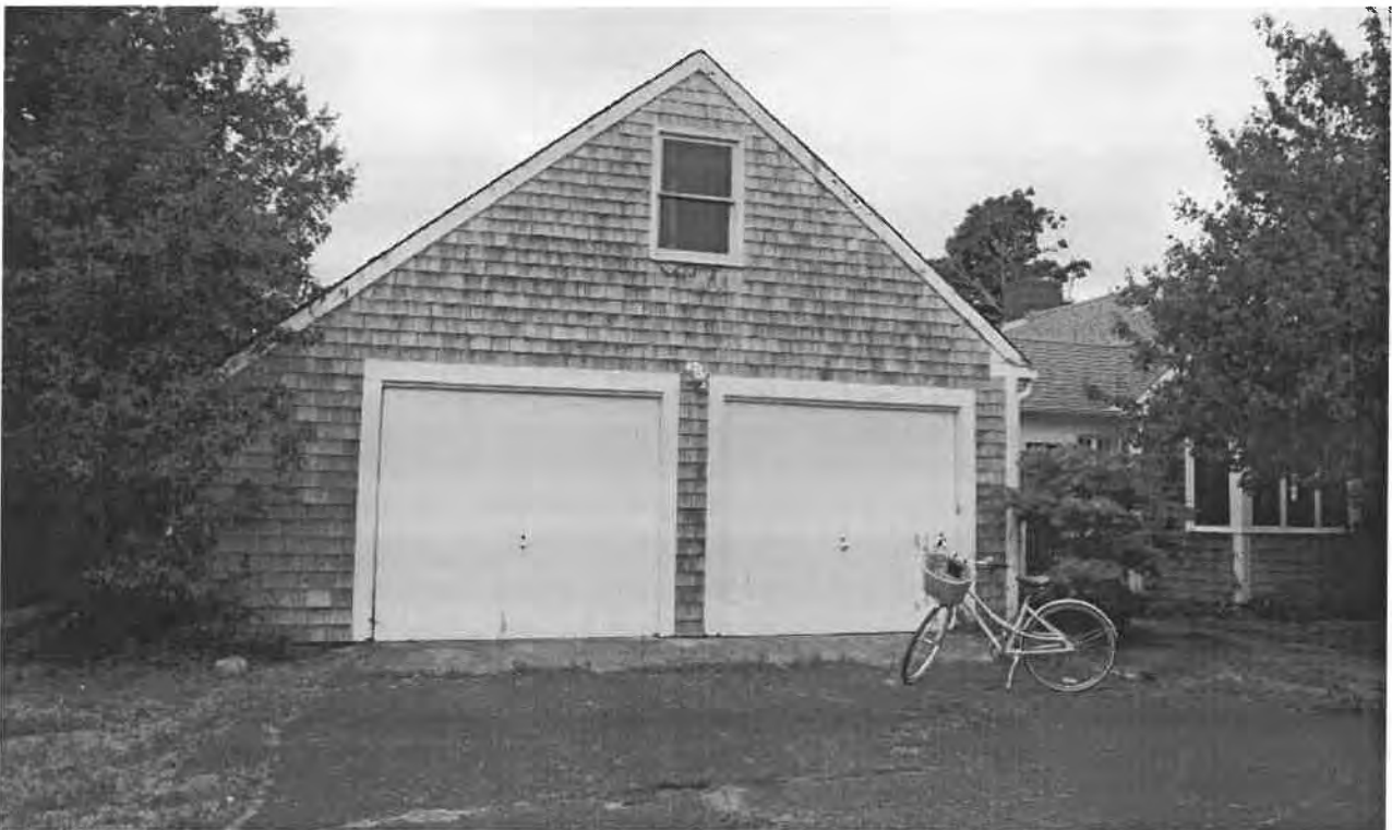
VIEW OF WEST ELEVATION (LEFT FROM FRONT)
