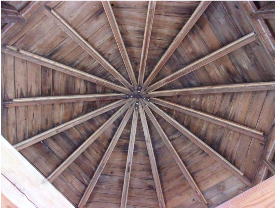
Typical existing (original) dome roof framing with visible water staining at third floor
