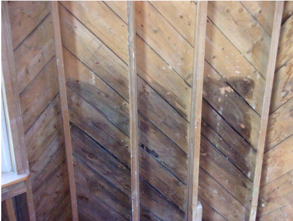
Typical third floor board sheathing with visible water staining and deterioration; constructed with dimensional lumber
