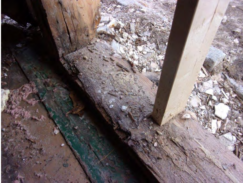
Typical deteriorated first floor sole plate at exterior wall (in contact with foundation); no mechanical fasteners connecting sole plate to foundation
