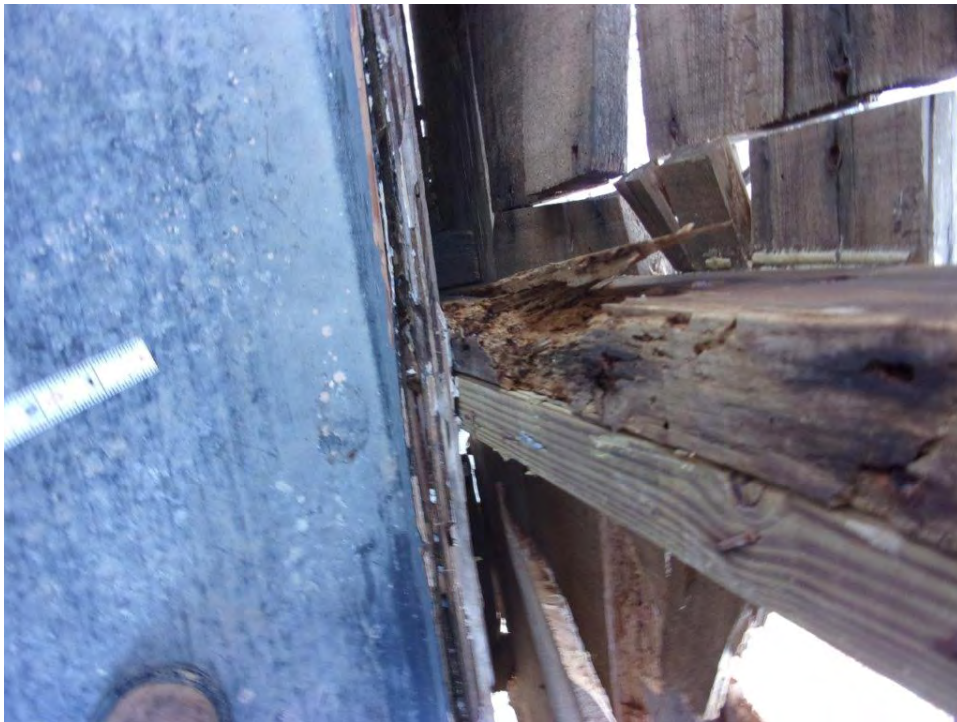
Typical rotted/deteriorated second floor wrap-around balcony board sheathing and exterior railing post; constructed with dimensional lumber
