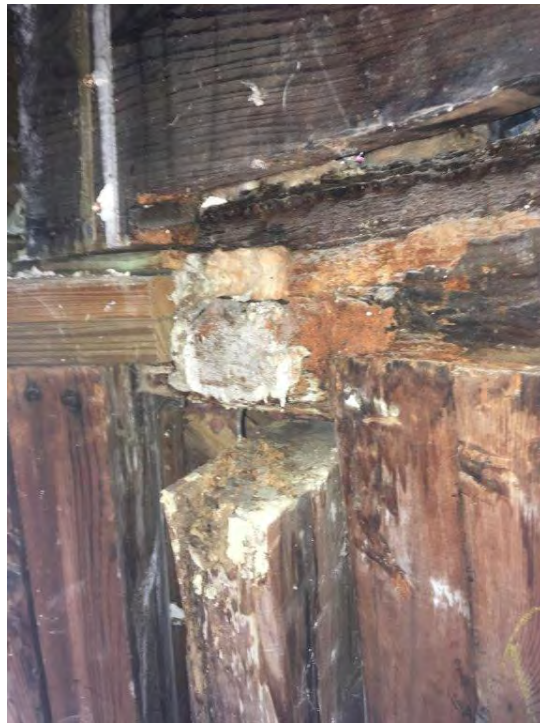
Typical second floor wall stud fully separated top plate; no longer providing support to gravity load resisting system
