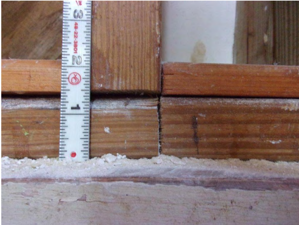
Typical discontinuous second floor exterior wall sole plate joint with no mechanical attachment observed
