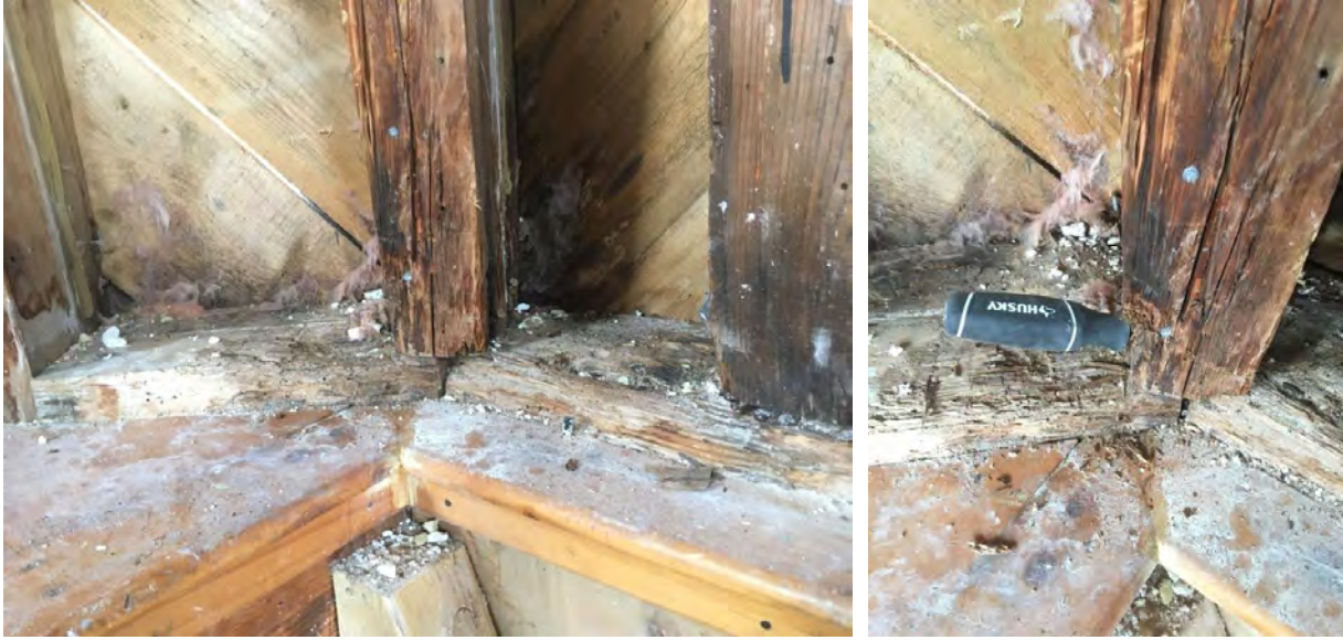
Typical second floor exterior wall stud rot/deterioration at sole plate of second floor exterior wall
