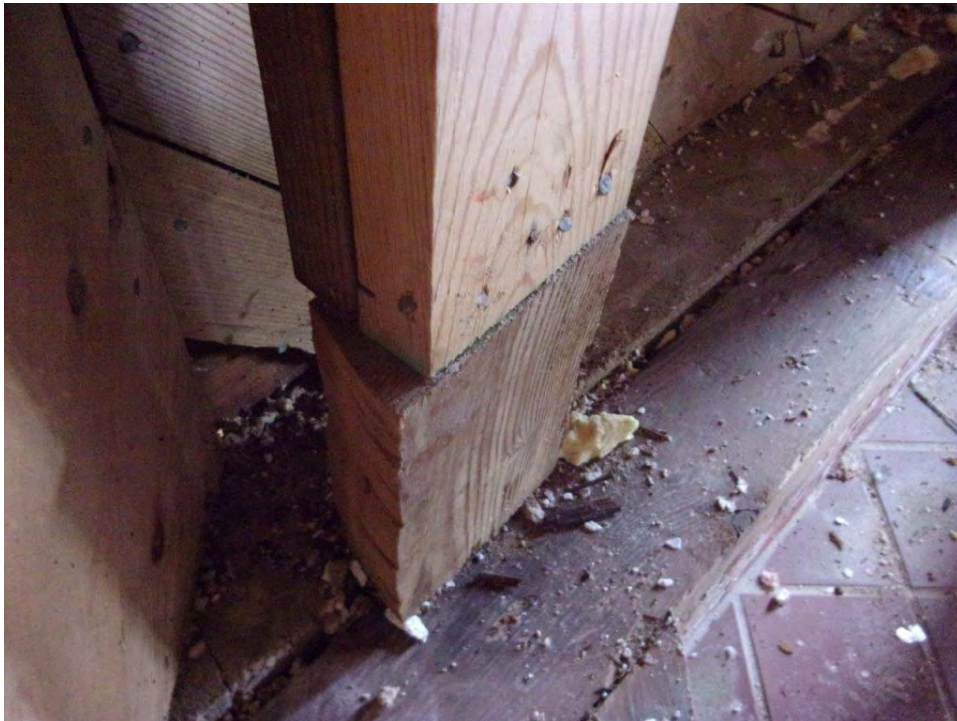
First floor supplemental framing with discontinuous column framing; no mechanical fasteners securing column base to foundation
