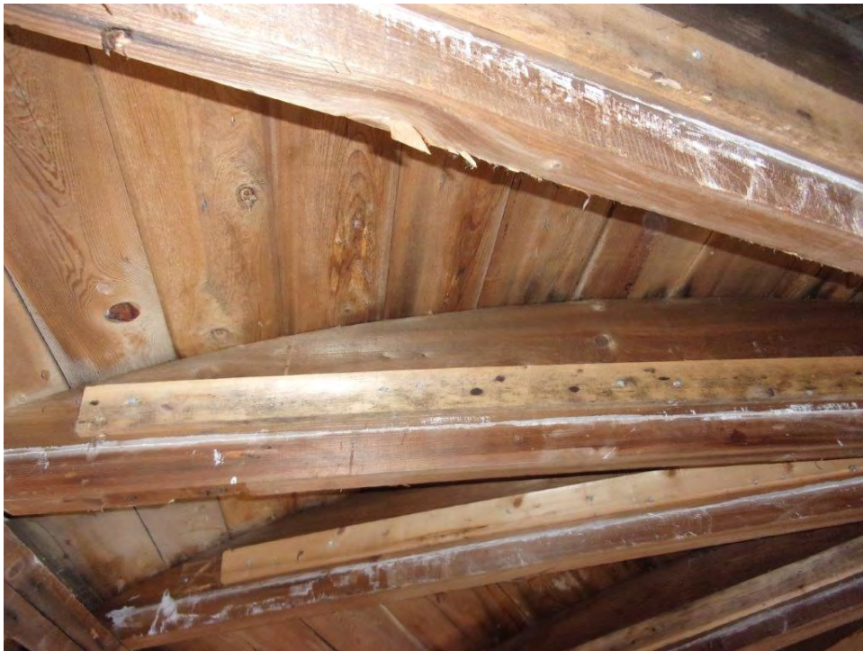
Typical dome roof framing curvature and board sheathing with visible signs of water staining
