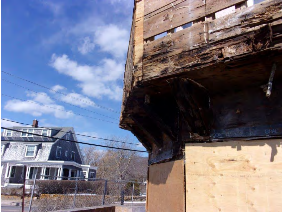
Typical second floor wrap-around balcony sheathing and supports; constructed with dimensional lumber
