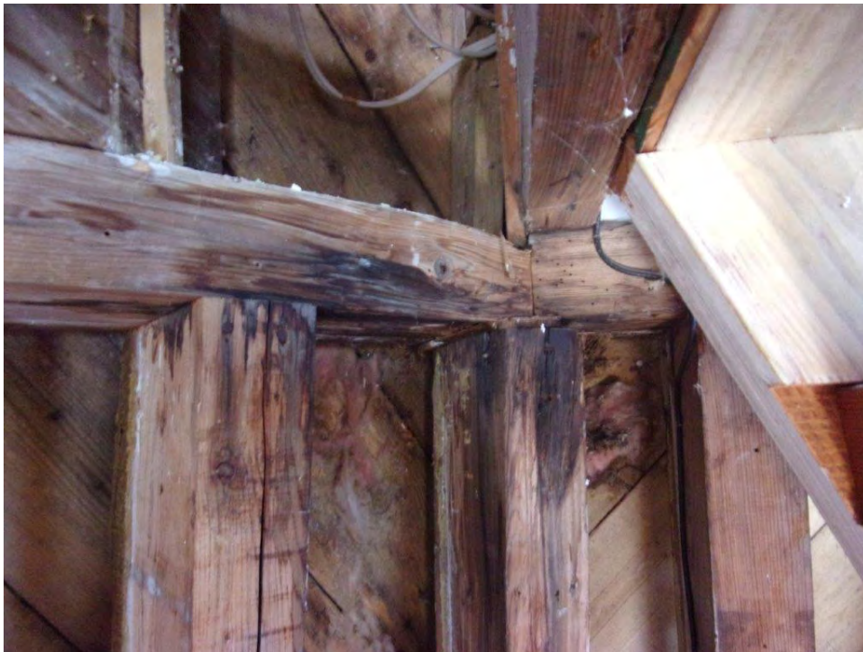
Second floor exterior wall framing with visible water staining, rot & crushing of top plate
