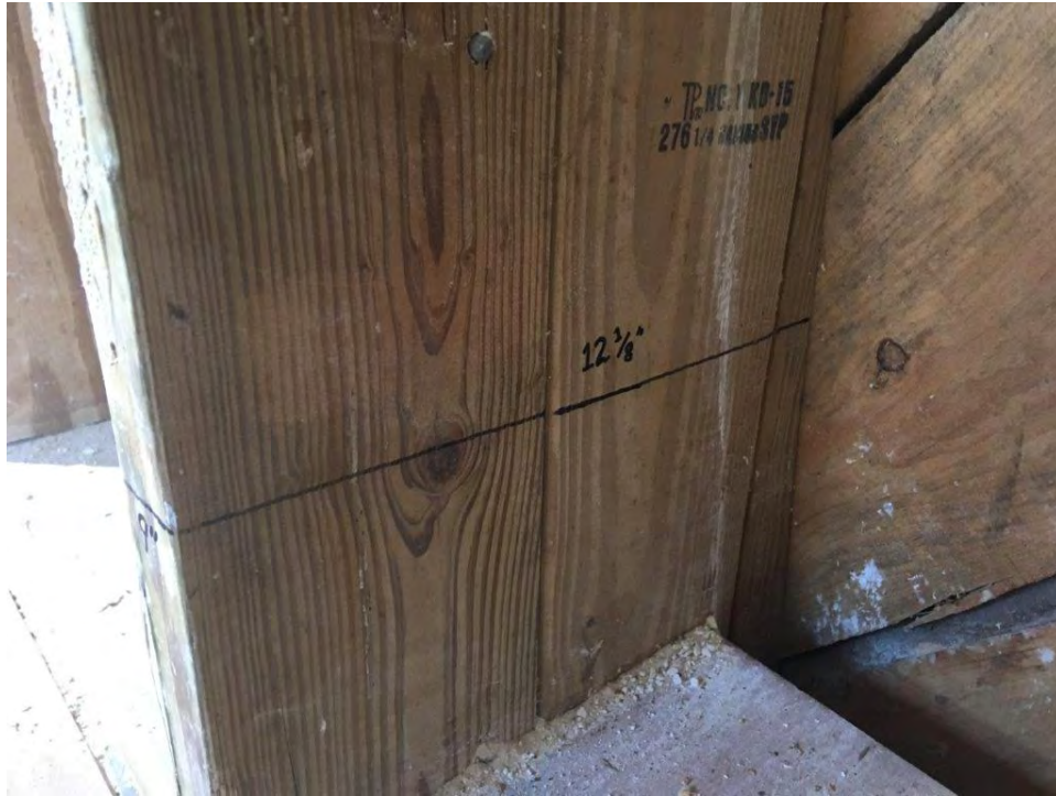
Typical third floor wall framing with “wedges” at exterior surface; “toe-nailed” mechanical attachment secured stud to wedge
