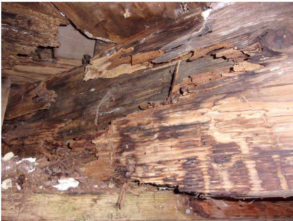
Typical deteriorated/rotted end of second floor support beam at first floor exterior wall top plate
