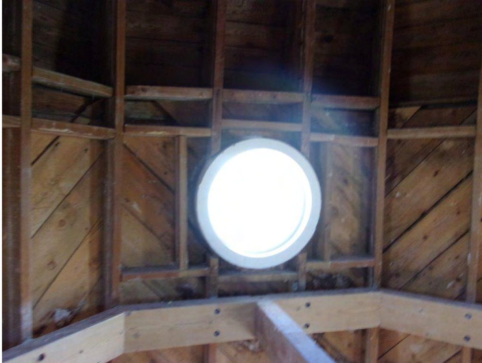
Typical third floor exterior wall framing at portal window; no jack or king studs installed (discontinuous gravity load path); constructed with dimensional lumber
