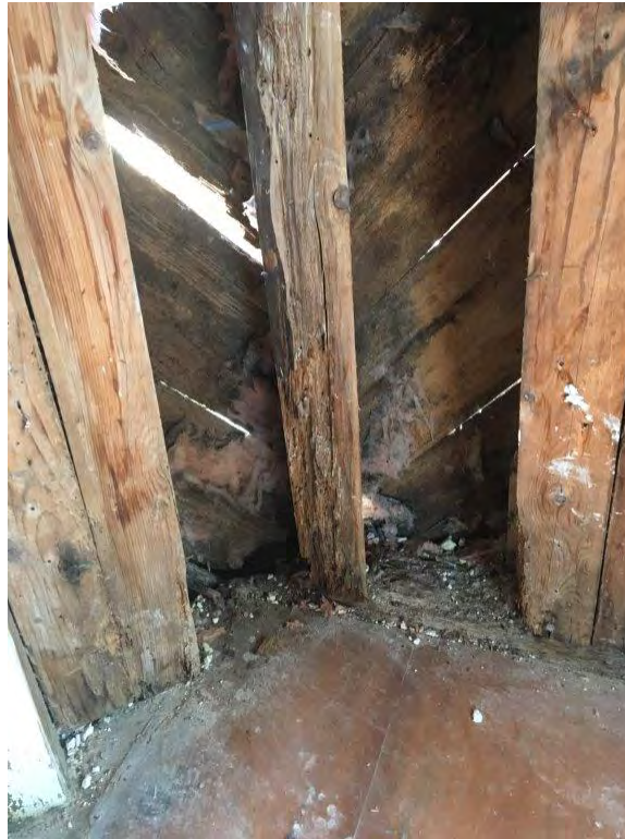
Typical second floor exterior wall stud and wall board with evidence of staining and deterioration
