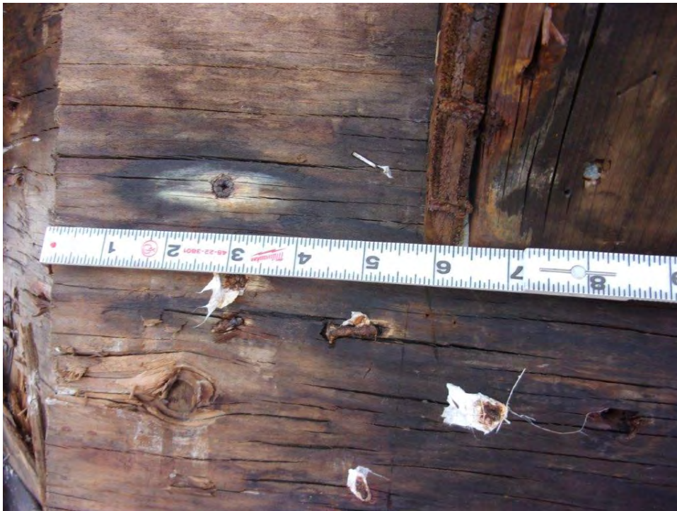
Typical second floor wrap-around balcony with separation of sheathing from diagonal support; constructed with dimensional lumber
