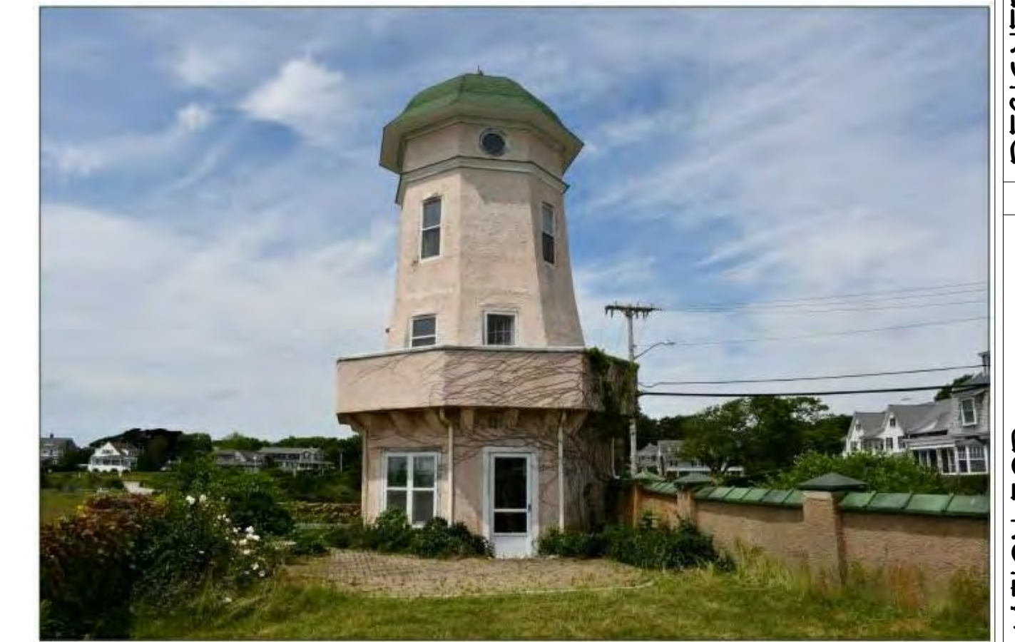
22. Lighthouse, facing west
