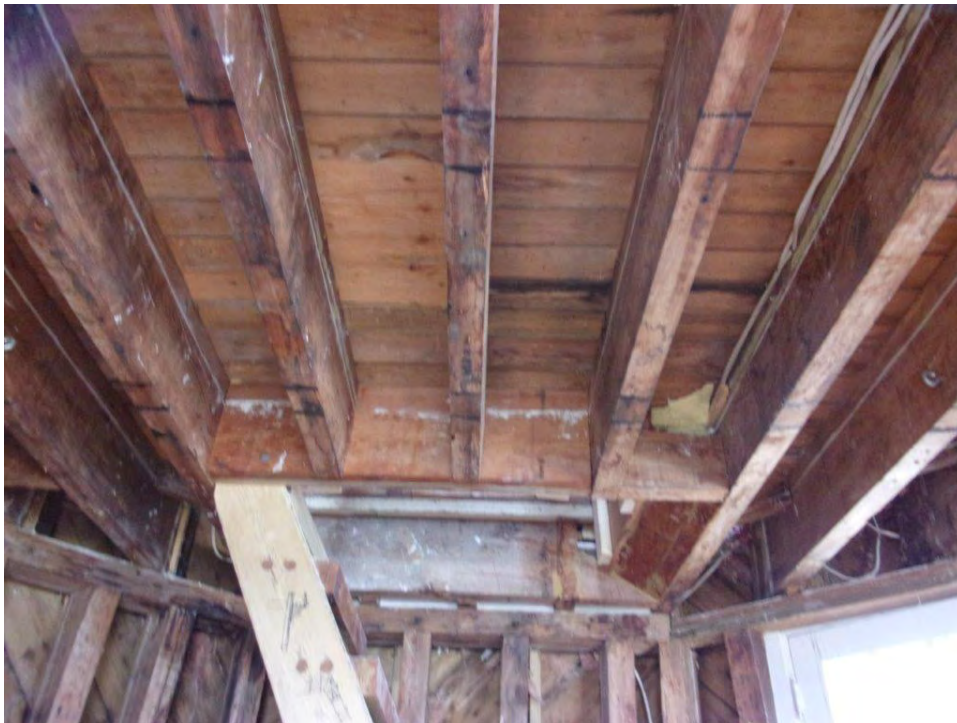
Typical third floor support framing with discontinuous header at stair opening framing at third floor
