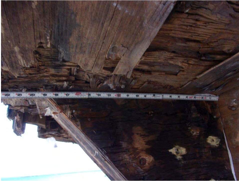
Typical underside of second floor wrap-around balcony with failed sheathing (layers separating); constructed with dimensional lumber
