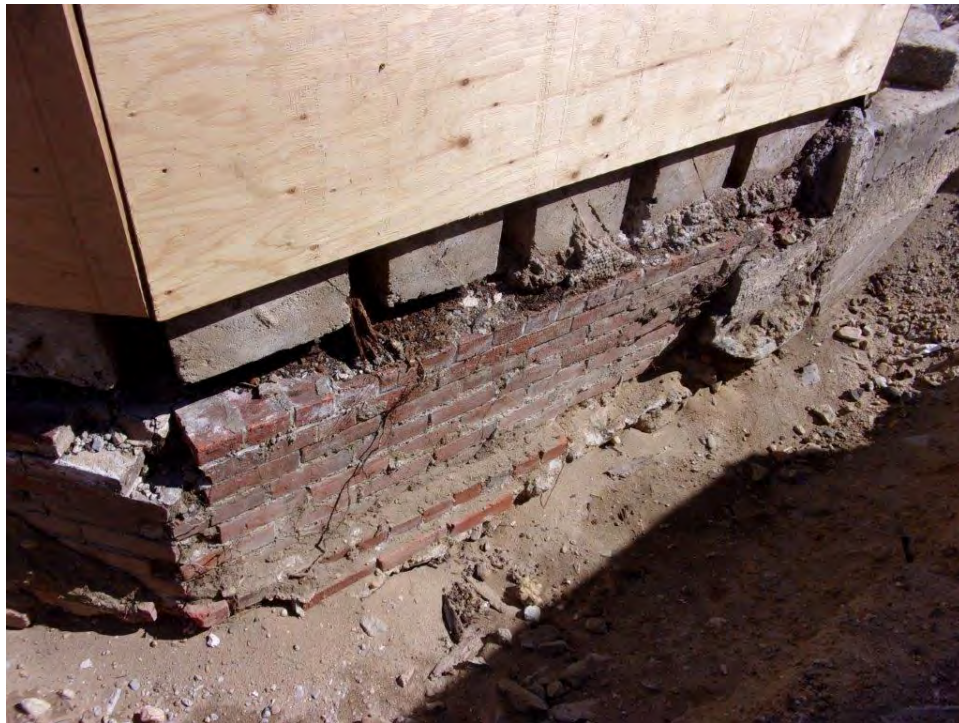
Typical building mass masonry and concrete foundation with concrete block installed between exterior wall studs; visible vegetative growth and deteriorated wood sole plate
