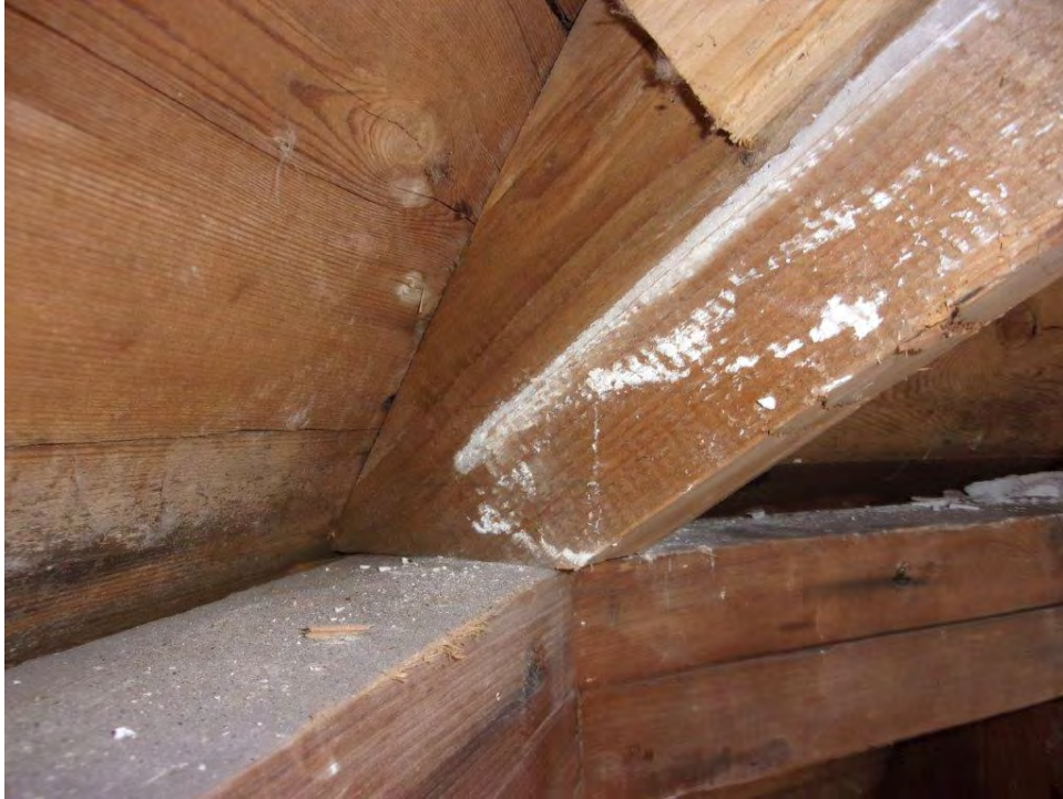
Typical dome roof framing support at double top plate at third floor exterior wall; no mechanical fasteners observed
