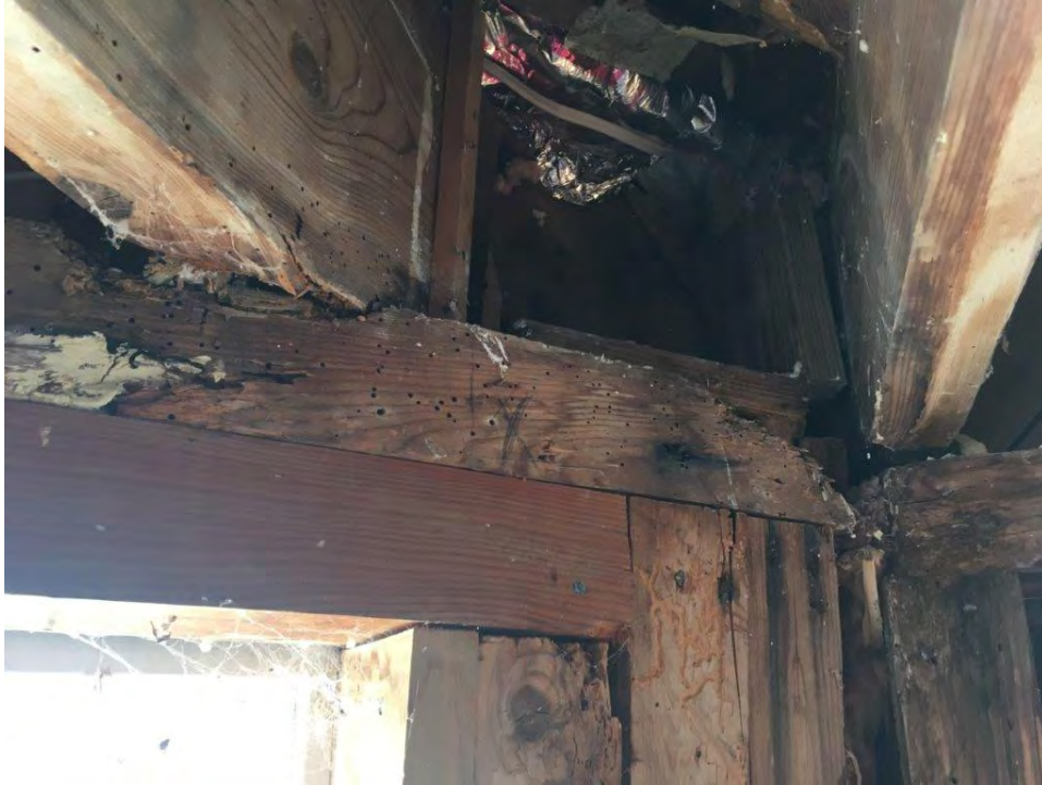
Third floor beam with evidence of insect infestation and bearing failure at second floor exterior wall top plate; deterioration/rotting visible along top plates
