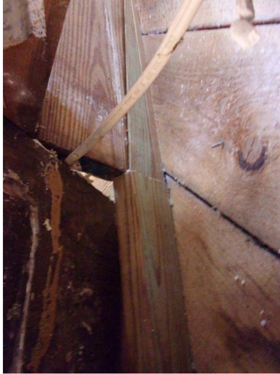
Typical third floor exterior wall stud and “wedge” not fully supported; mechanical fastening of wedges to studs not observed
