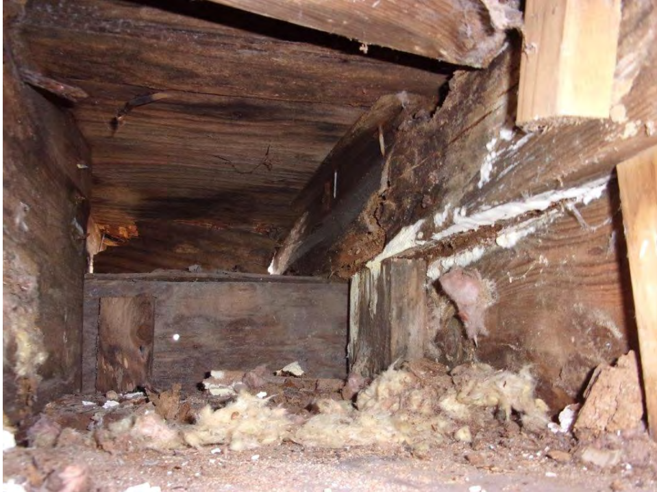
Typical deteriorated cantilever support beam for wrap-around exterior balcony at first floor exterior wall top plate (underside)
