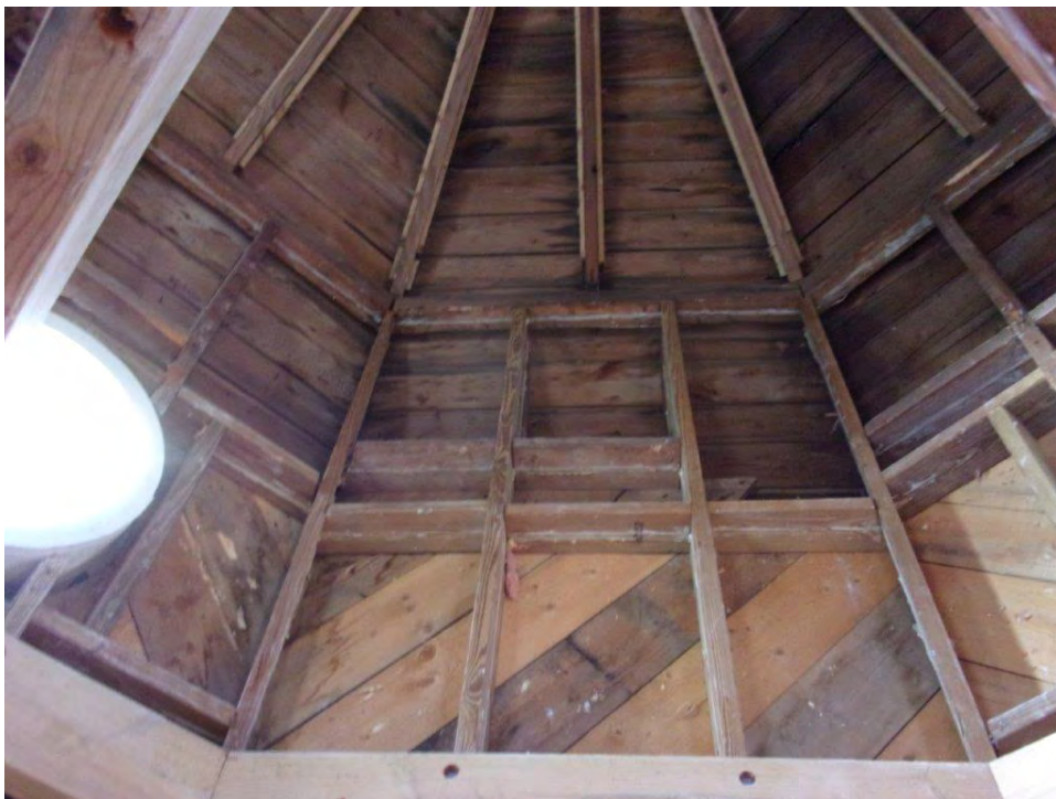
Visible discontinuous bridging at dome roof eave at third floor exterior wall framing
