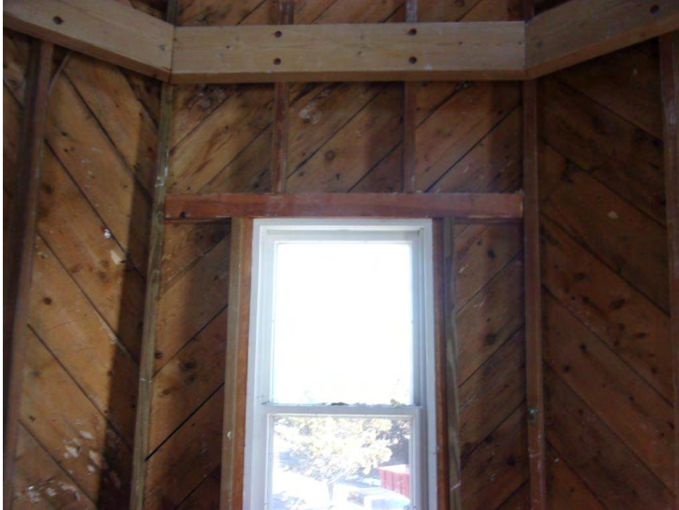
Typical third floor window header and tension/compression ring wood framing; tension/compression ring framing secured with carbon steel fasteners
