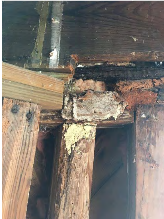
Rotted/deteriorated steel plate and wood top plate installed at second floor exterior wall
