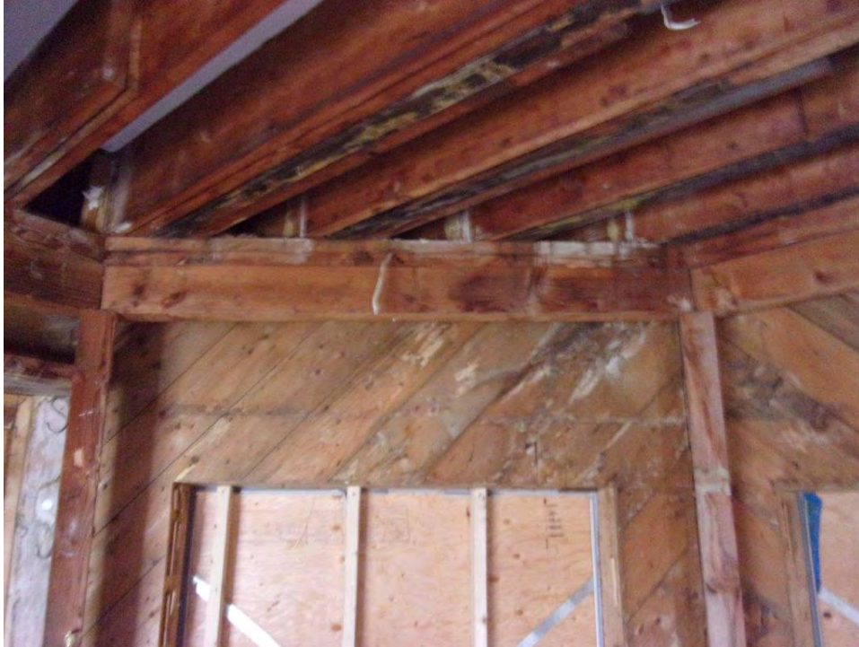
Typical second floor supplemental support framing with sporadically fastened, sistered floor beams; no mechanical fasteners connecting supplement interior framing
