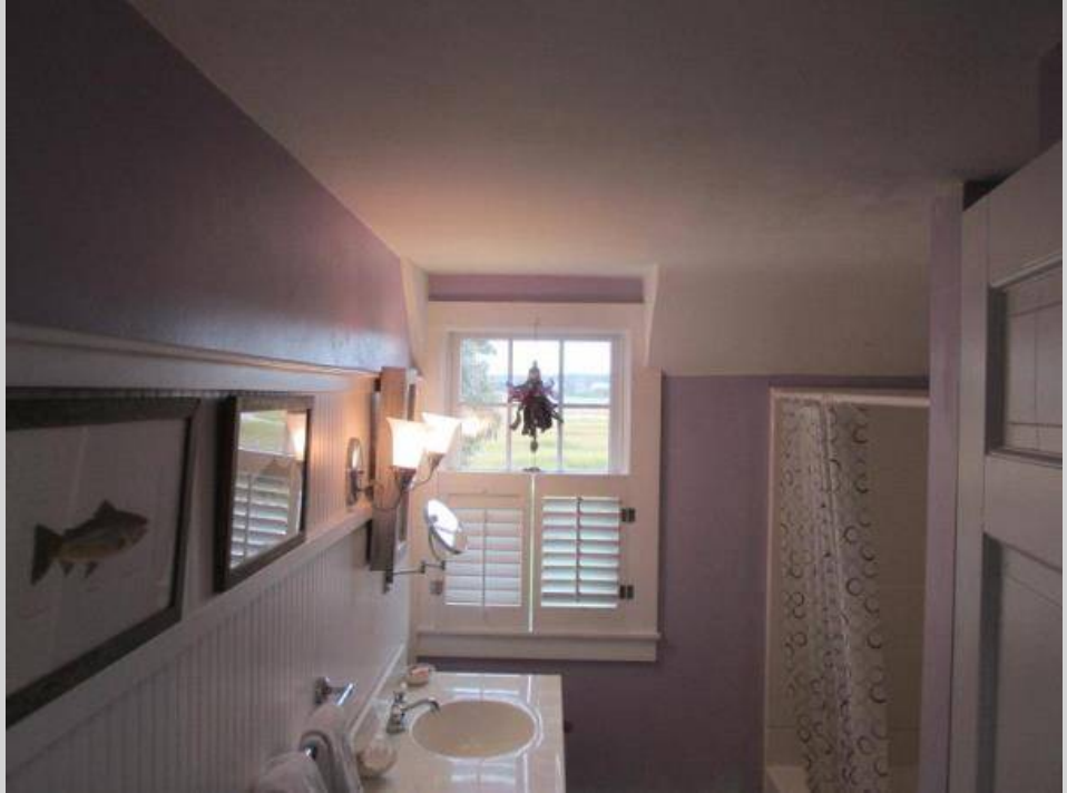
There is a window and fan for bathroom ventilation. ** FUNCTIONAL ventilation.
