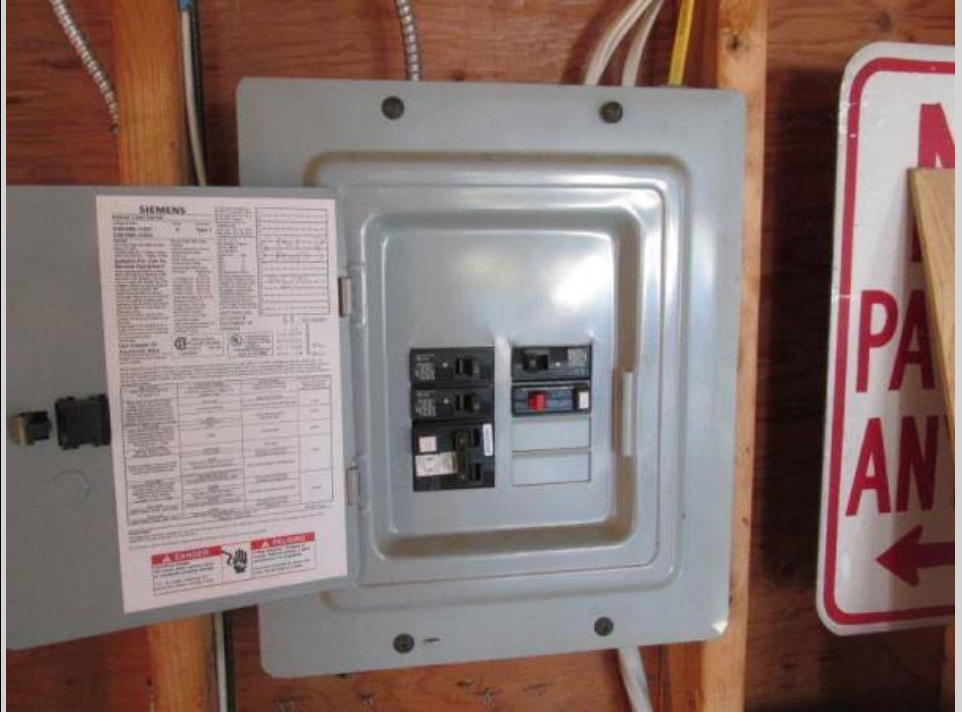
A sub panel, powered from the main panel is located in the garage.
