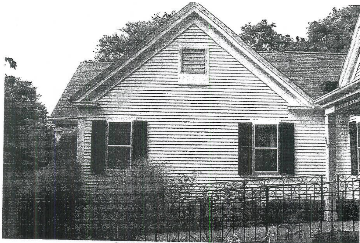
South Side, showing Addition (1962)
