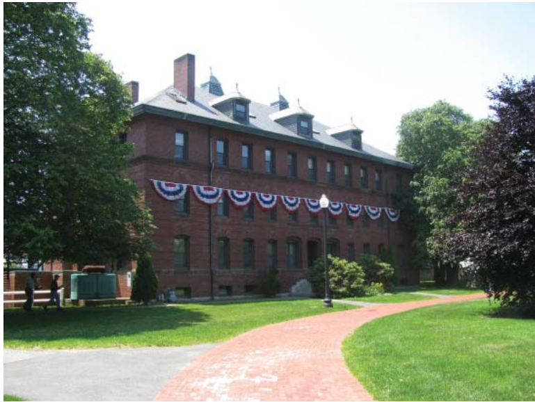
Town Hall Building, Hyannis. Photo by Community Opportunities Group, Inc.
