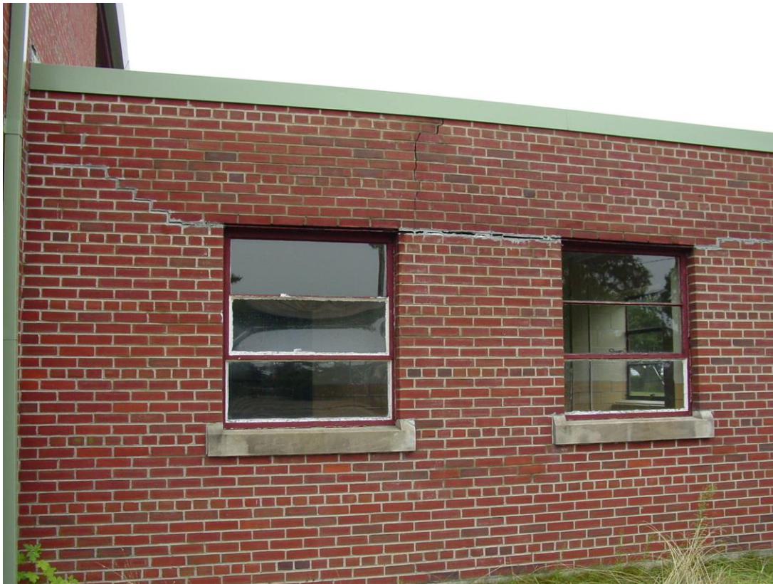
Figure 2. Masonry damage caused by failing steel lintels
