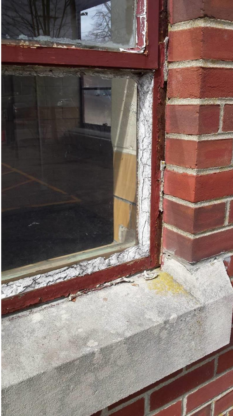
Figure 3. Typical damaged metal window with asbestos caulking
